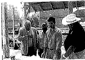
Review In-progress Construction
