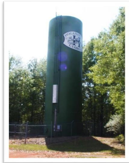
Pine Street Standpipe (100,000 gallons)
