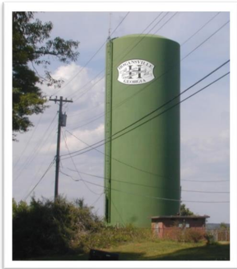
Granite Street Standpipe (175,000 gallons)
