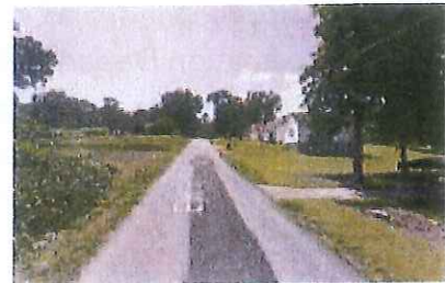
Looking west on Elm Street
