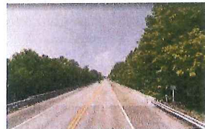
Bridge at Yellow Jacket Creek
