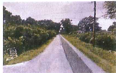
Looking west on Elm Street
