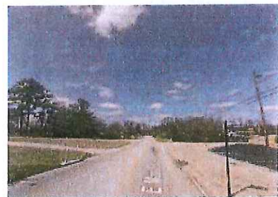
East Main Street near Lincoln Street (looking west)
